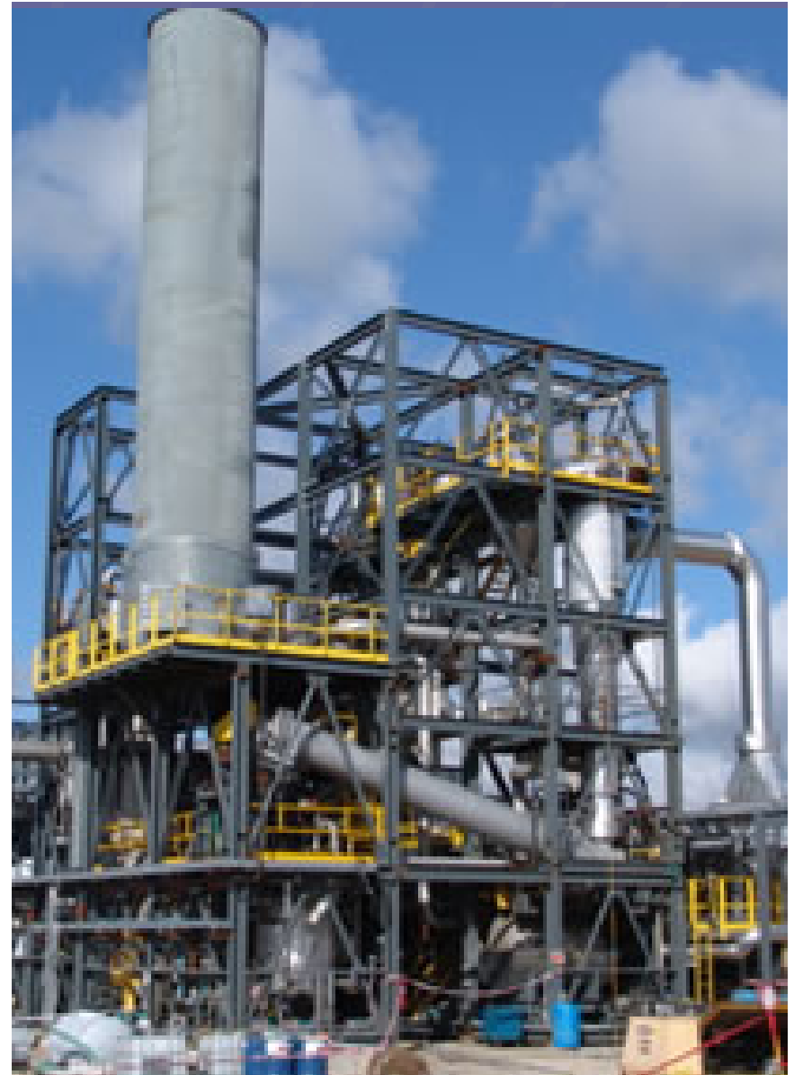
Modern Fast Pyrolyzer Dynamotive Energy Systems Co. 200 dry ton/Day plant West Loren Ontario CA
